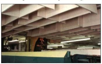
Figure 36. Sound-Absorption Paneling
