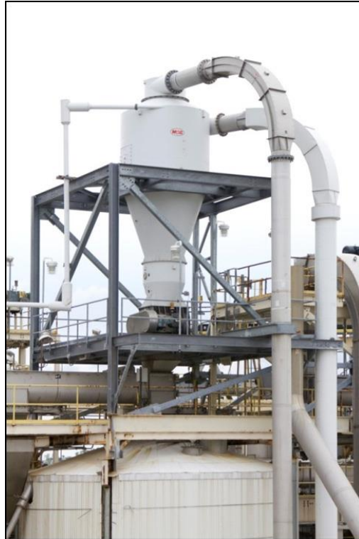
Figure III.4 Air Material Separator (Cyclone)
