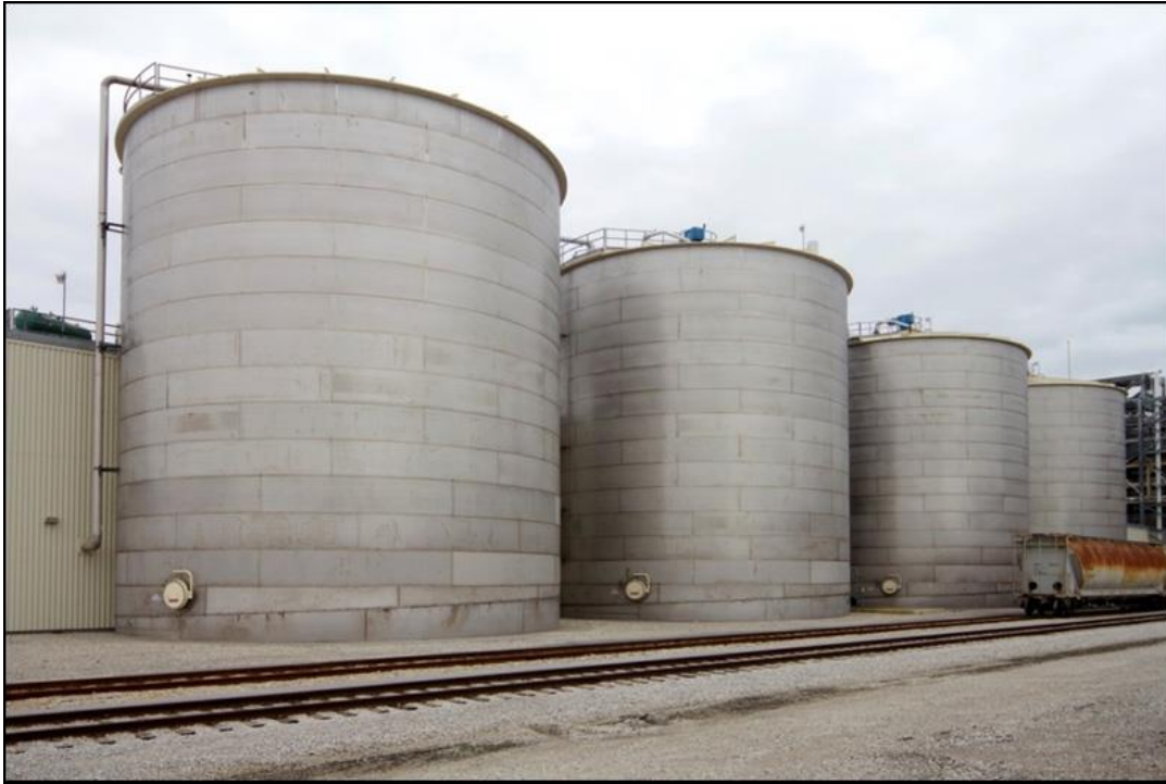
Figure II.12 Ethanol Fermentation Tanks
