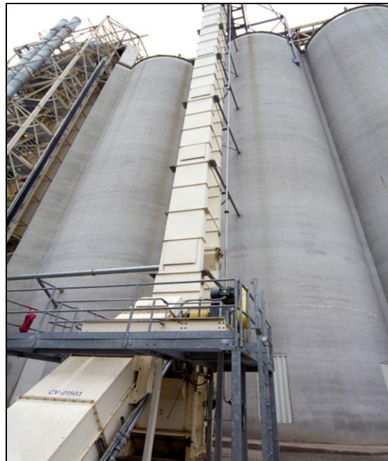
Figure II.9 Bucket Elevator and Storage Silo
