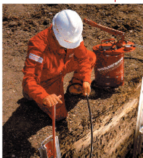
PHOTO: Speedshoring Corporation Vertical shore
