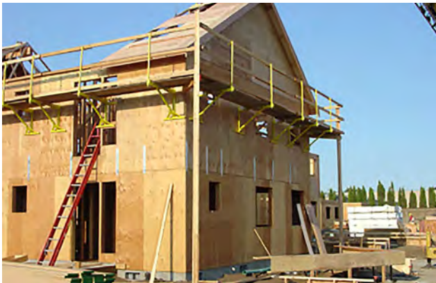
Manufactured exterior carpenter's bracket scaffolding.
