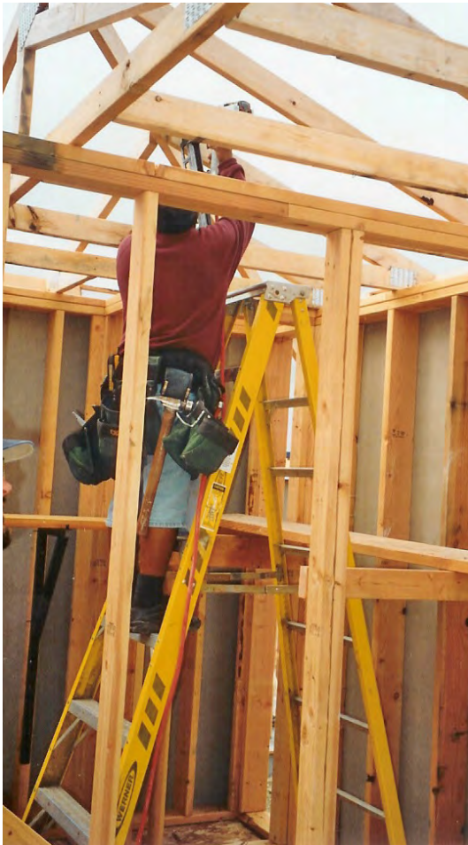
Working at the peak from the top plate of an interior wall.
