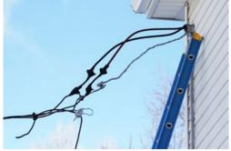
branch?" When placing a non-self-supporting ladder against an upper support, be mindful that both side rails must equally rest against the upper-support surface unless the ladder (or ladder's approved accessory) is designed for a single point of contact. For all ladders, electrical hazards are easy to overlook. Check before you raise your ladder. Finally, consider the weather. Is there hazardous weather such as ice, high wind, or electrical storms that can affect the ladder's safe use?
