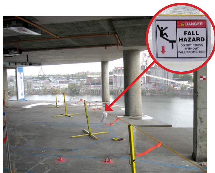
A warning line must be set up so it eliminates the risk of a worker falling over the edge. Use signs and flagging to emphasize the hazard.
