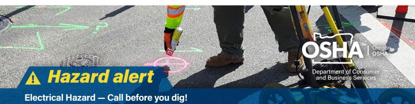
An incident in Oregon involved an apprentice electrician who was driving an eight-foot grounding rod for a temporary electrical service. The rod was about four feet into the ground when it struck an energized underground conductor.
