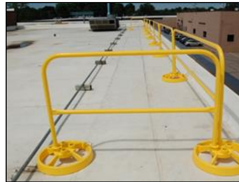
Figure 3. Temporary guardrails
