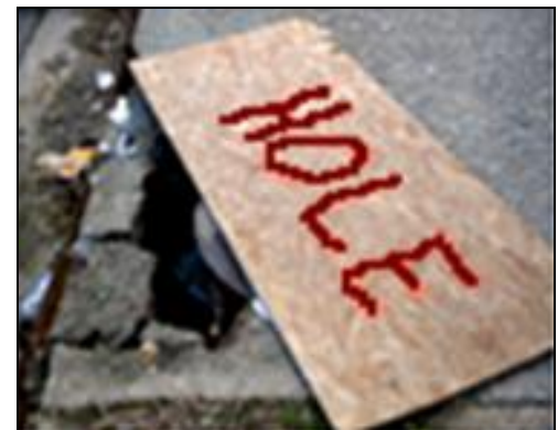
Figure 9. Plywood hole cover
