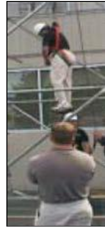
Figure 17. Worker suspended in harness prior to rescue
