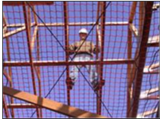
Figure 13. Safety net system
