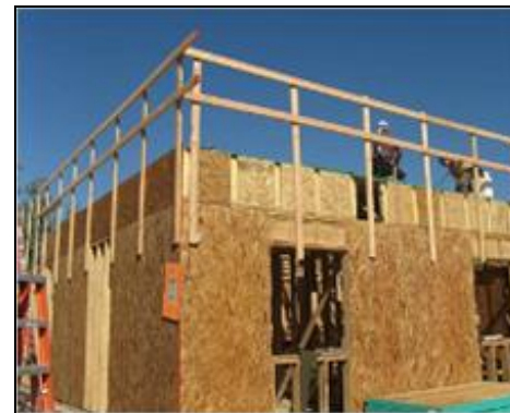
Figure 4. Temporary guardrails
