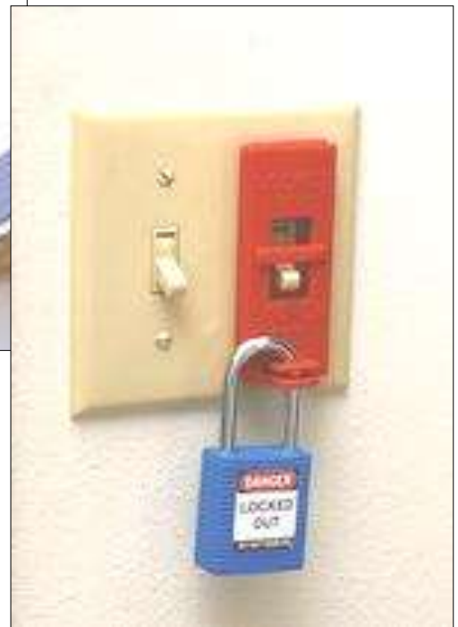
Wall switch lockout
