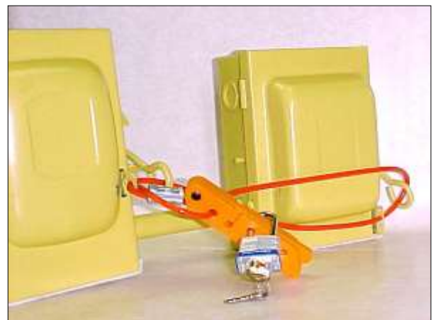
Two electric boxes locked out
