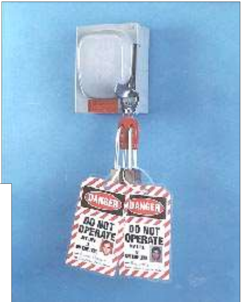
Multiple lockout using a multiple lockout hasp
