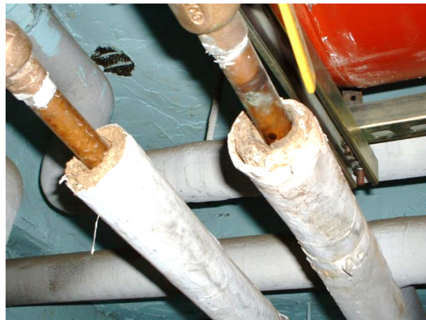
Asbestos wrapped pipes. The pipe on the right shows damage which can cause asbestos fibers to go airborne.
