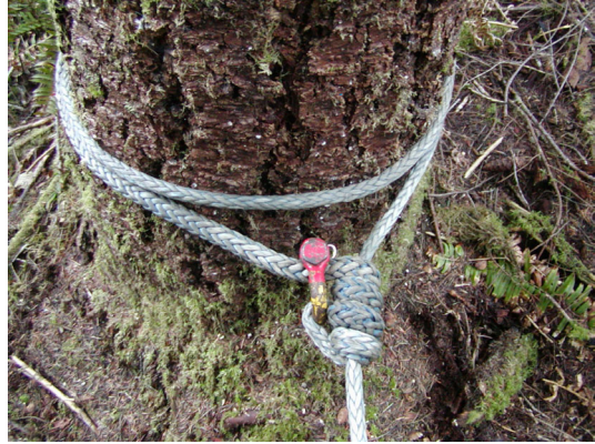
Figure 3. Termination of guyline with shackle
