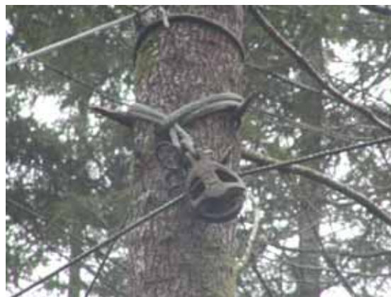
Figure 6. Synthetic tree strap, endless loop design
