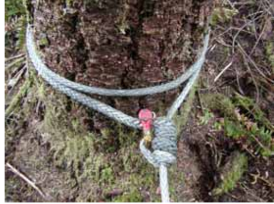
Figure 3. Termination of guyline with shackle
