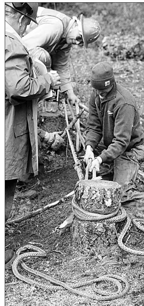
WORKING TO TIGHTEN a "woopie sling" of Am-Steel Blue synthetic rope is one of the crew members with the help of Steve Pilkerton.
