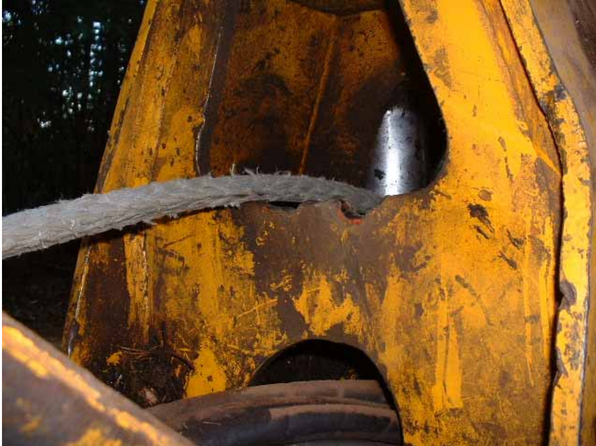
Figure R13. Grooves shown are cut in 1/2-inch steel plate by wire rope under improper operation of fairlead arch. Abrasive surfaces such as this must be dressed smoothly prior to use of synthetics. Synthetic rope will not stand the abuses that steel wire rope will. Continued operation in this mode will create undue shortening of operational life of synthetic rope due to fraying of fibers and resultant reduction in rope strength.
