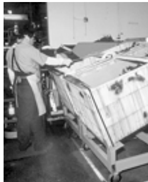
Tilted container with step for easier access
