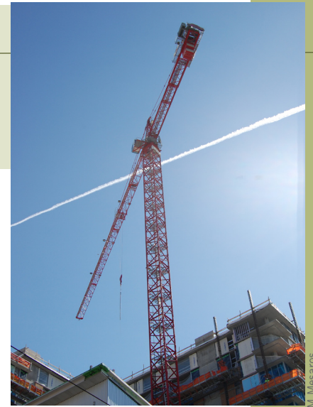
Crane at work in northwest Portland
