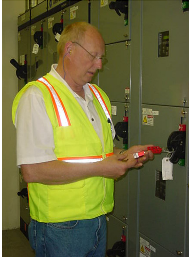
Ron Richardson adjusts a lockout/tagout system.
