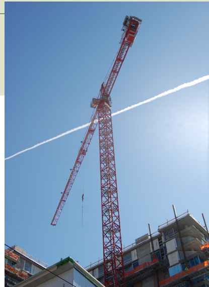
Tower crane at work in northwest Portland
