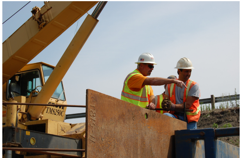
Dave Parsons works with a contractor on an ODOT excavation project in Portland.
