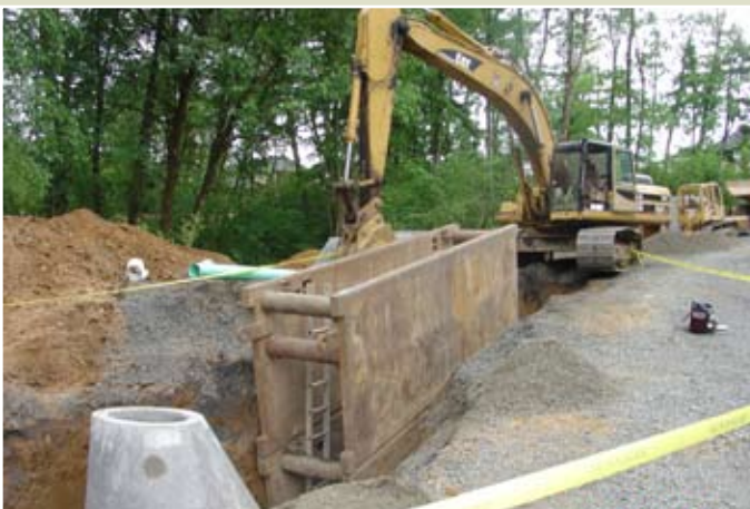
The hook and shackle broke loose and went through the shield, striking the worker in the head.
