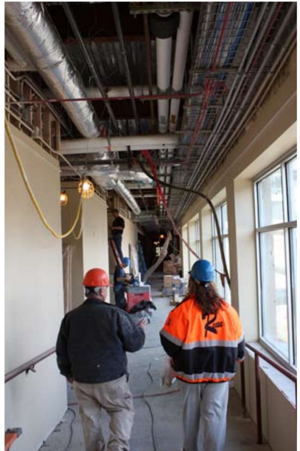
Electrician Brian Gilfillan talks with Shelley Nasby about some of the job challenges at the Newport site.
