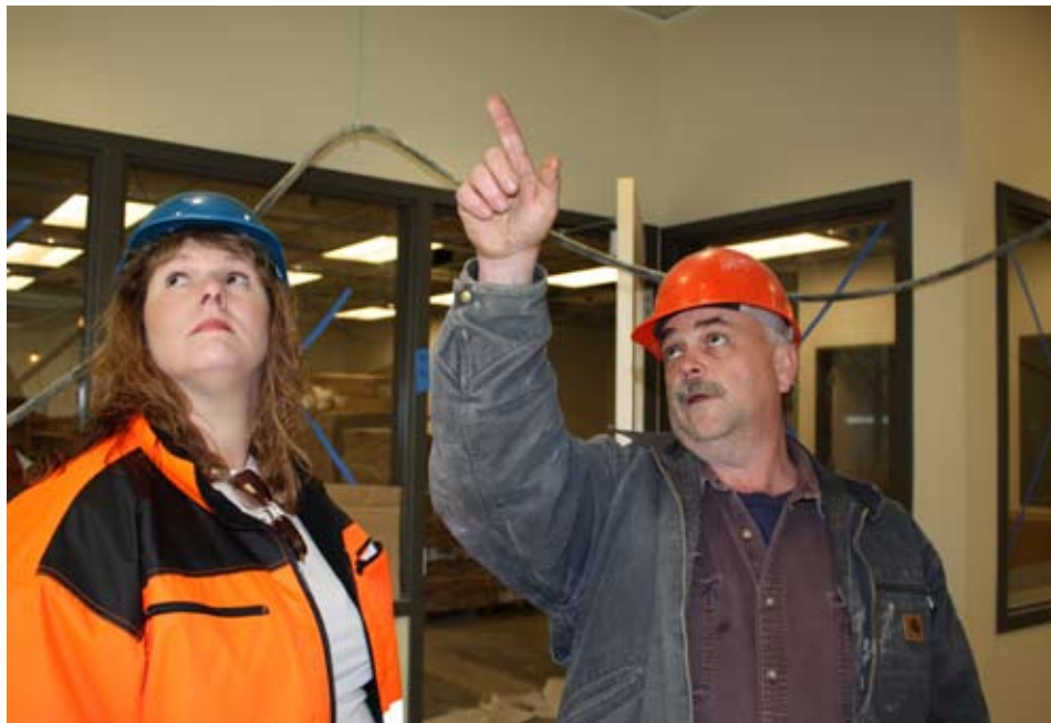
Shelley Nasby conducts a review of a jobsite in Newport with electrician Brian Gilfillan.
