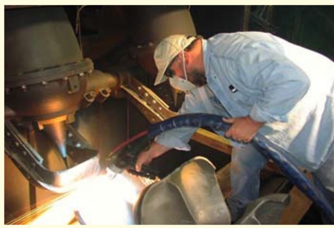
Dan Becker performs the thermal spray equipment demonstration. While Dan applied the coating at the plant in Bellingham, Wash., he was videotaped so the process could later be shown in a sales video.
