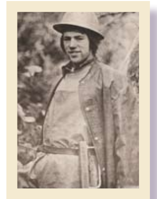
Ralph’s son, Tim Huffman, the rigging slinger, working with the rigging crew.
