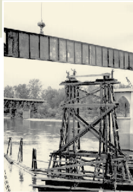
Construction of Marion Street bridge across the Willamette River, Salem, Ore. Workmen are waiting on scaffolding to place the first steel girder being lowered into place in the construction of the Marion Street bridge in 1952.
