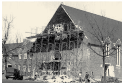
Construction of the First Christian Church in Salem, Ore., 1951. Scaffolding can be seen on the front end, as workers install the rose window. The photo is from the Hugh Stryker Collection.
