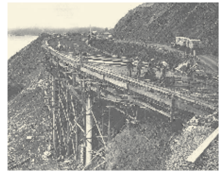
Construction of Rocky Point Bridge on Oregon coast highway, 1950.
