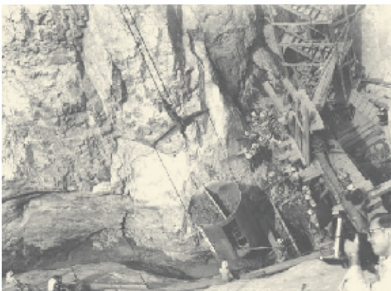
Construction of Detroit Dam on the North Santiam River in Marion County, Ore., 1950. Detroit Dam, a 463-foot high concrete gravity structure, is built on the North Santiam River about 47 miles east of Salem.
