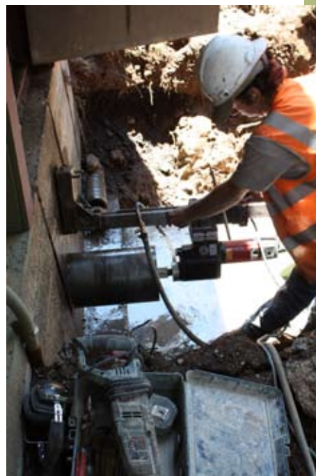
Wade Haury of We Cut Concrete drills into concrete for a heating pipe at Pilot Butte Middle School in Bend.
