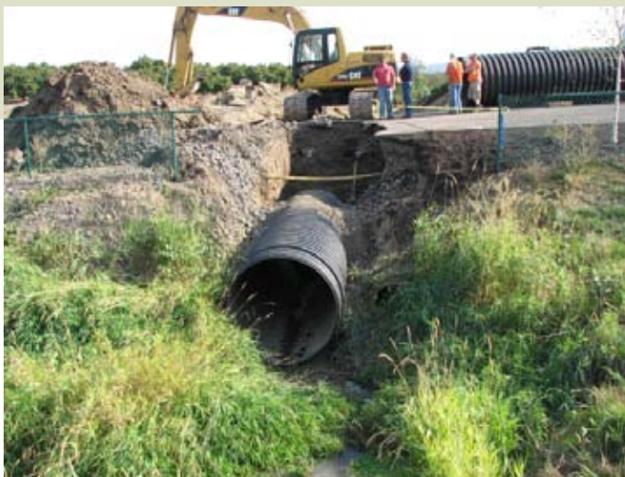
A crew member was trapped when the above trench collapsed between the pipe and track-hoe.
