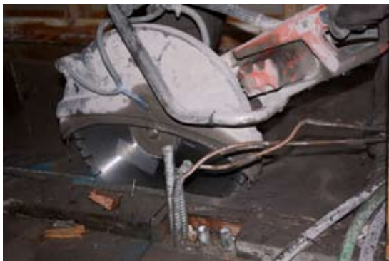
We Cut Concrete uses wet saws during nearly every job.
