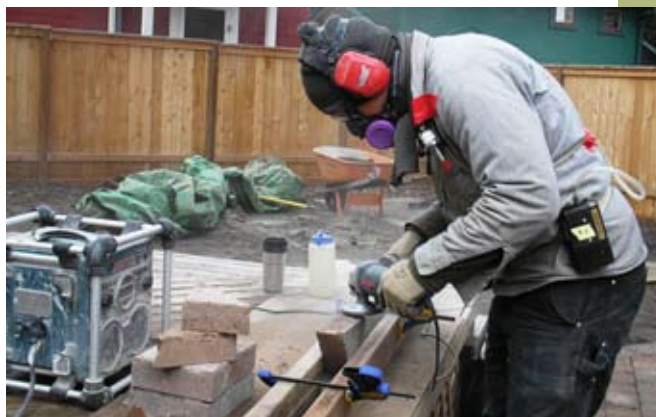
A worker grinding brick was overexposed to silica at this Portland site. (Photo: Lori Cohen, Oregon OSHA, Portland)
