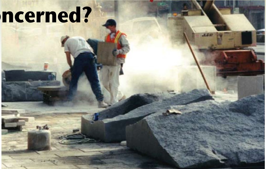
Sampling showed this masonry contractor in Medford, working with concrete block, was overexposed. (Photo: Tim Capley, Oregon OSHA, Medford)
