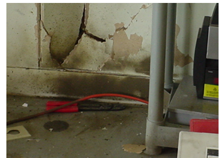
Damage to wall near compressor
