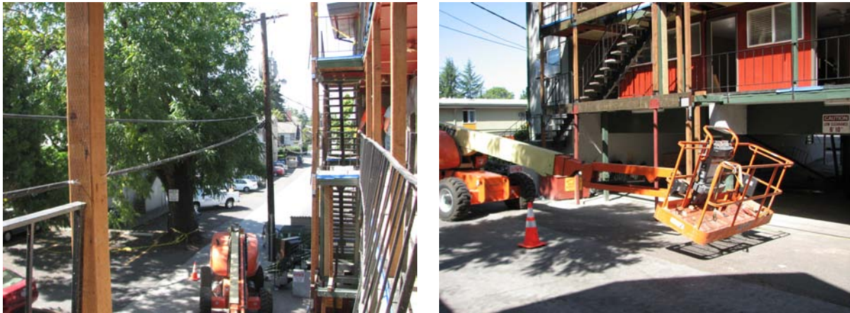
The distance between the apartment complex and the high-voltage wires was estimated to be six feet. The aerial platform was eight feet by four feet.
