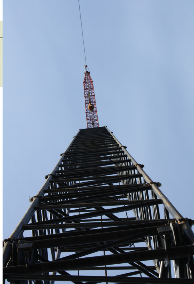
A view from below one of Hamilton Construction's cranes.
