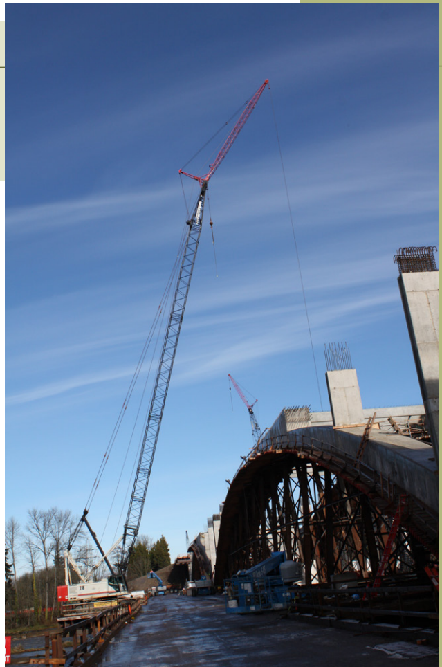
Several cranes coordinate picks on the I-5 bridge project in Eugene.
