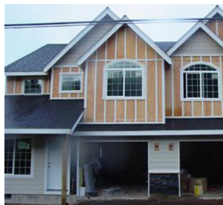
The residence and the power line.
