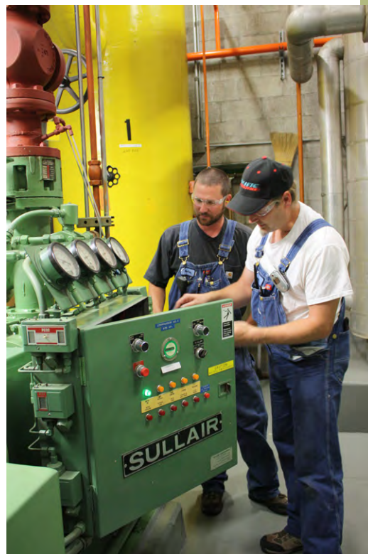
Nathan Duckwall (left) and John Nagy are in charge of maintaining the company’s ammonia system.
