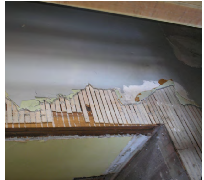
Asbestos was discovered during a 2011 home remodel in Portland. (Photo: Chris Zimmer)
