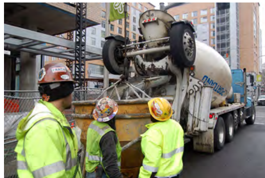
Top left: Potter and Jeremy Freeman inspect chains of crane hook. Top right: The building is constructed in close proximity to the craftsman style home in the foreground. Bottom right: Crane work on 17-story building on the Portland State University campus. Bottom middle: Bryan Ware, Jeremy Freeman, and Potter watch for crane hook to pick up the concrete bucket. Bottom left: Jason Trickett works on rebar.
