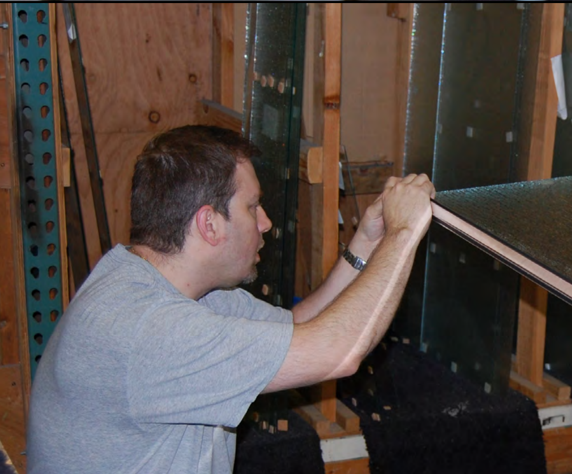
Chris White installs a frame to a glass door.
