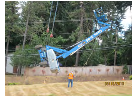
Right: A crane was used to remove the lift following the accident..
