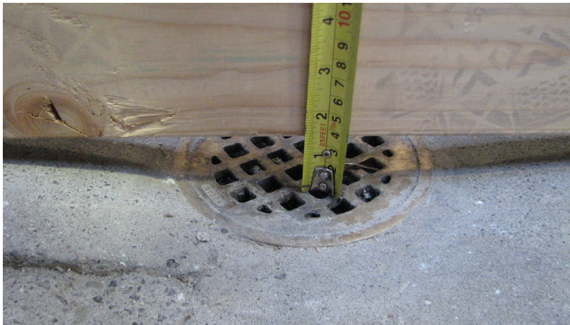
One of the two drain holes in the floor was 1½ inches below the surface.
