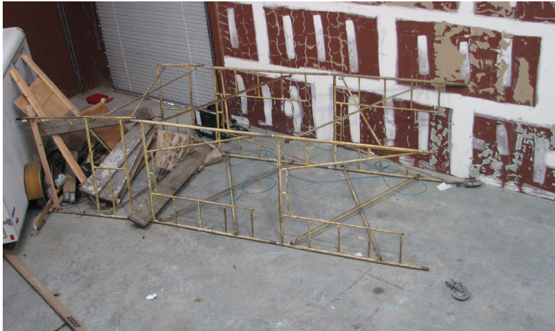
Loose casters and an uneven floor led to the scaffold tipping over.
