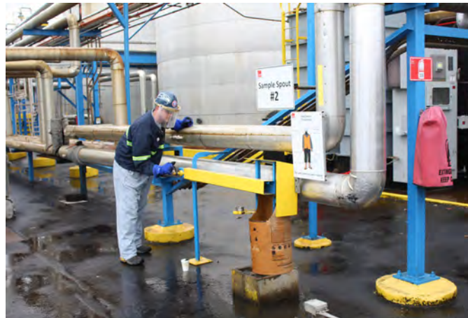
Above: A remote valve opener was installed to increase distance and decrease exposure to asphalt splash and fume hazards. Kyle Halpin takes several samples each day for quality control. Left: A contractor wears PPE while cleaning out an asphalt tank.
