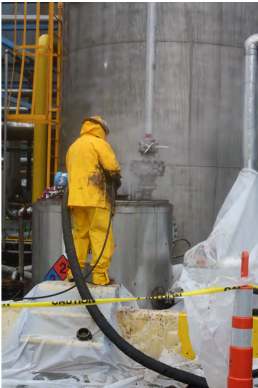
Above: A remote valve opener was installed to increase distance and decrease exposure to asphalt splash and fume hazards. Kyle Halpin takes several samples each day for quality control. Left: A contractor wears PPE while cleaning out an asphalt tank.
