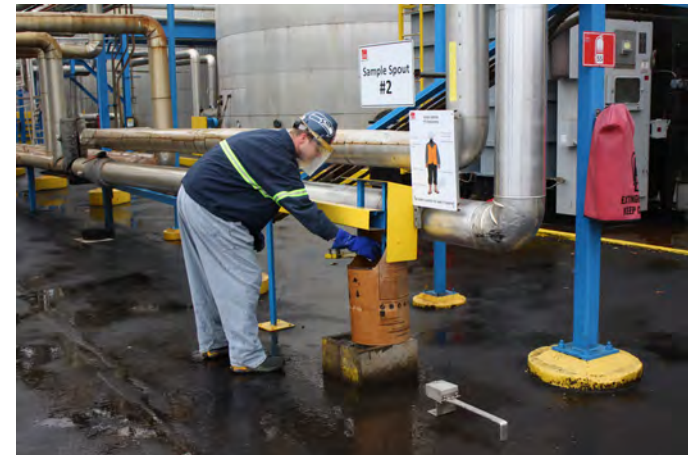
Above: A remote valve opener was installed to increase distance and decrease exposure to asphalt splash and fume hazards. Kyle Halpin takes several samples each day for quality control. Left: A contractor wears PPE while cleaning out an asphalt tank.
