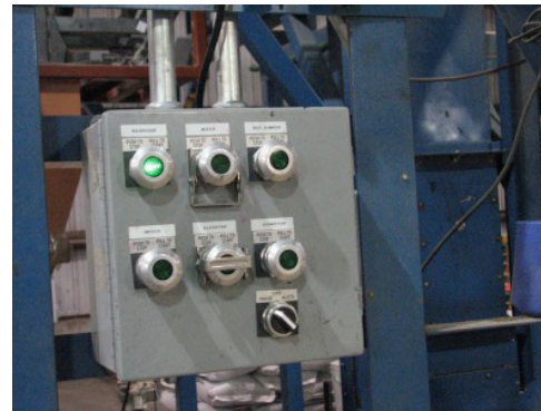
The conveyor control switch and mixer control.
