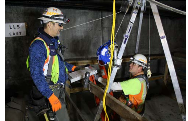
Hoffman Construction has already implemented changes to be in compliance with Oregon OSHA's new confined space standard.
