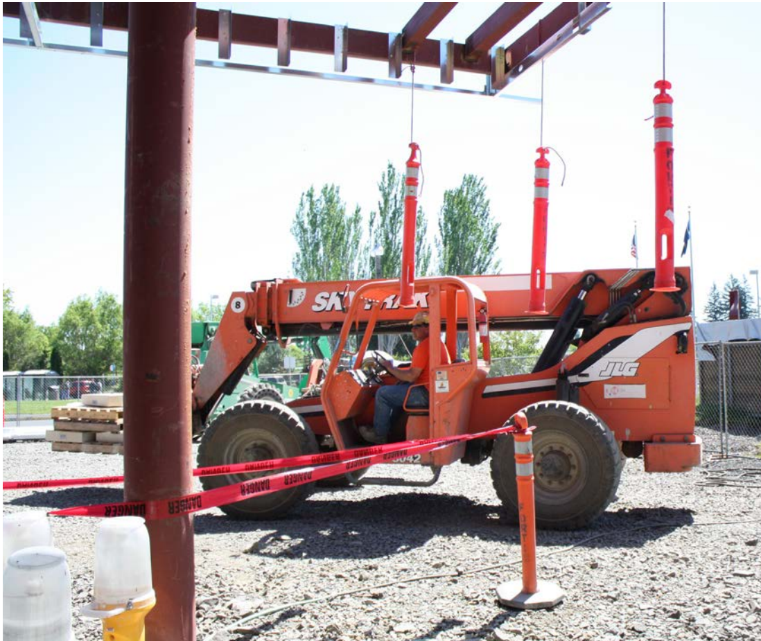
Hanging cones help guide construction traffic from coming too close to a building in progress on the Rock Creek campus of Portland Community College.
