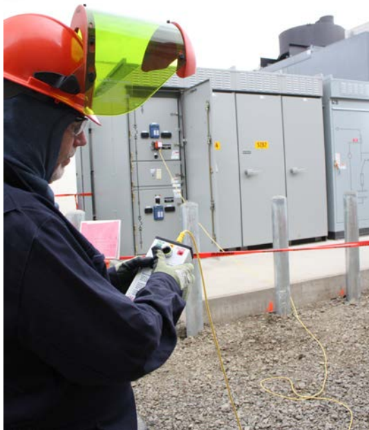
Chuck McCarty (left) of Rosendin Electric uses a Chicken Switch (remote control) to test a 12.47kV medium voltage switch gear at a data center project. Workers can control breakers from outside the arc flash zone. Arc flash protective clothing is not necessary because of the remote activation and other Fortis staff were clear of any danger.
