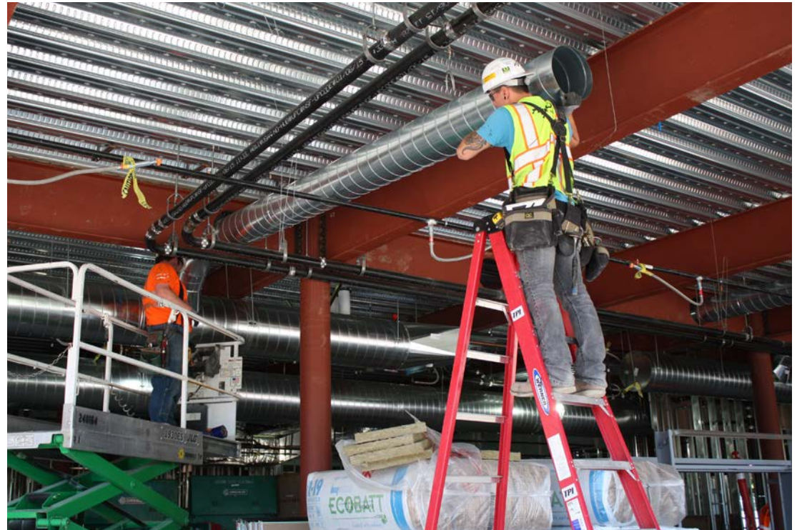
Workers from Apollo Sheet Metal install an HVAC system on a Fortis job. Star said sequencing work and pre-task planning help minimize risks during projects with multiple subcontractors.
