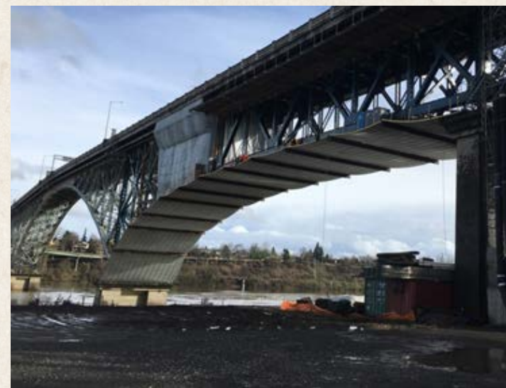
A worker who fell from an upper platform underneath the Ross Island Bridge was not protected by a fall protection system.
