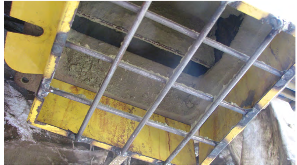
The guard that the company put over the housing after the incident.
