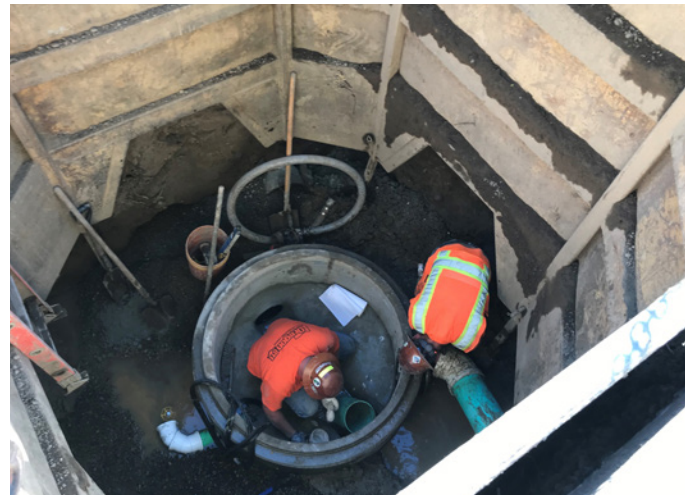
Two employees in excavation making pipe connections.
