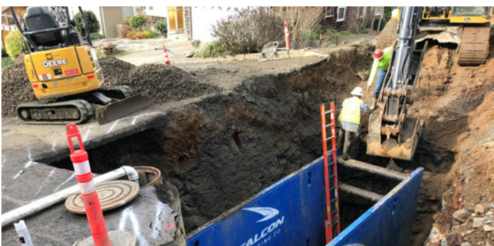
Unsafe egress. Employee egressing from trench had no choice but to have help to get out safely. Foreman is the person with the red hard hat helping out employee egressing.
