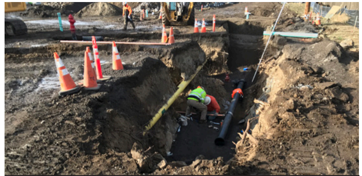
Excavation is not sloped at an angle no steeper than one and one-half horizontal to one vertical (34 degrees measured from the horizontal).
