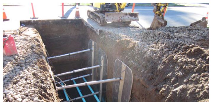
Protective shoring system did not extend to the top of the excavation.
