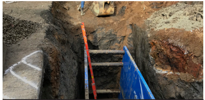
Protective shoring system did not extend to the top of the excavation. Also, no cave-in protection at the open end of the trench box.
