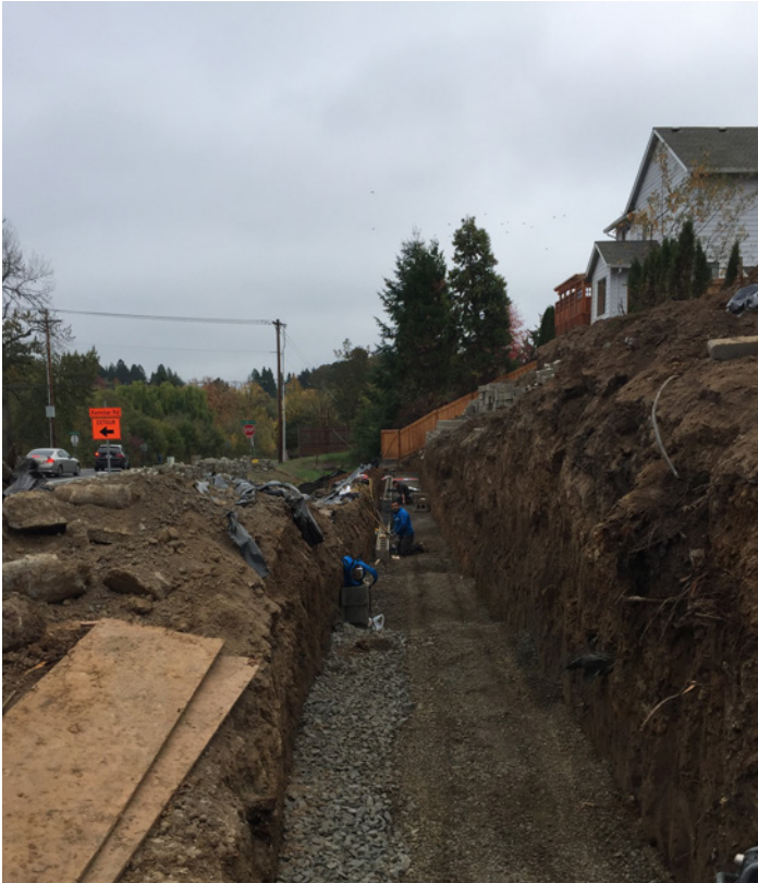
Two workers are exposed to a cave-in hazard while building a retaining wall next to a face cut. This illustrates that not just utility workers can be exposed to excavation/cave-in hazards, and that employers need to evaluate work areas and recognize cave-in hazards.
