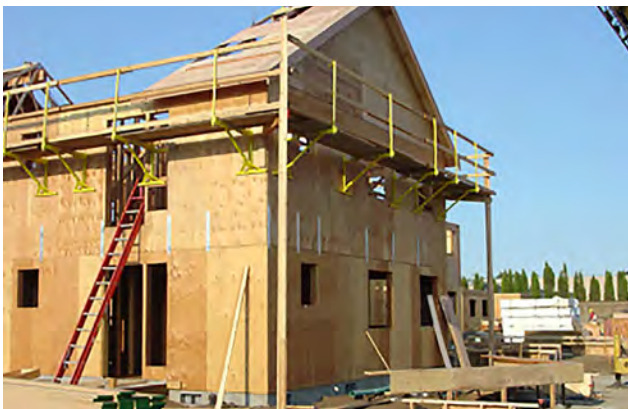
Manufactured exterior carpenter's bracket scaffolding.
