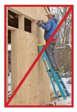
Standard stepladder used in a nonapproved configuration
