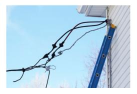
branch?" When placing a non-self-supporting ladder against an upper support, be mindful that both side rails must equally rest against the upper-support surface unless the ladder (or ladder's approved accessory) is designed for a single point of contact. For all ladders, electrical hazards are easy to overlook. Check before you raise your ladder. Finally, consider the weather. Is there hazardous weather such as ice, high wind, or electrical storms that can affect the ladder's safe use?
