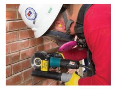
Full and proper implementation of dust collection systems on handheld grinders must meet all of the following:
