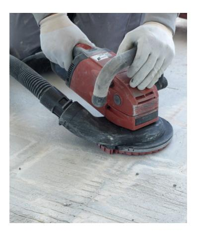
Cyclonic pre-separators and filter-cleaning mechanisms improve the suction of dust collection systems by preventing debris from building up on the filter. The grinder must be operated and maintained in accordance with manufacturer's instructions to minimize dust emissions.
