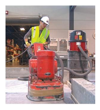
Option 2: Use a dust collection system recommended by the milling machine or floor grinder manufacturer, a filter with 99 percent or greater efficiency, and a filter-cleaning mechanism.
