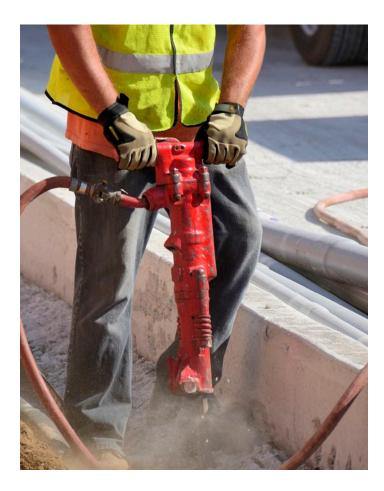
Jackhammers and handheld powered chipping tools must be operated with either a water delivery system that supplies a continuous stream of water at the point of impact, or a tool equipped with a commercially available shroud and vacuum dust collection system. Jackhammers and other handheld powered chipping tools must be operated and maintained in accordance with manufacturer's instructions to minimize dust.
