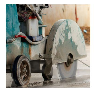
Walk-behind saws used to cut roads and cut pavement are typically used outdoors, though they can also be used indoors to cut concrete floors. When your employees use walk-behind saws indoors or in enclosed areas, you must provide additional exhaust to minimize visible airborne dust.
