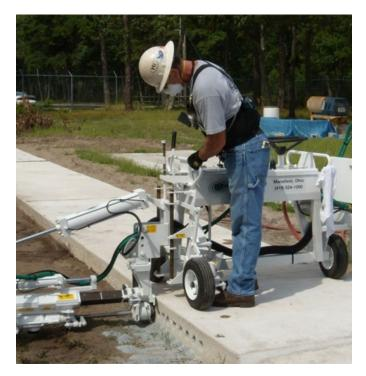
A HEPA-filtered vacuum must be used to clean holes. Compressed air can be used to clean holes when used in conjunction with a HEPA-filtered vacuum to capture the dust, or a hole cleaning kit designed for use with compressed air.
