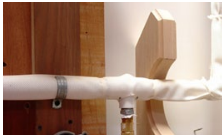
PVC pipe is prohibited in above-ground systems unless it is completely enclosed. Photo credit: Owen Smith, Oregon OSHA
