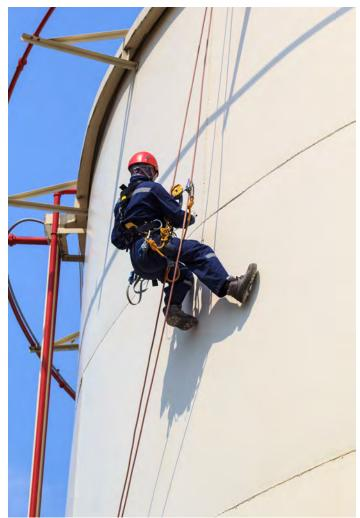
The building owner must inform the employer in writing that each permanent anchorage has been identified, tested, certified, and maintained so it can support at least 5,000 pounds in any direction.
