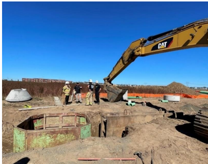
The excavation site, showing the excavator, the two trench shields, and the unprotected 30-inch gap between them.
