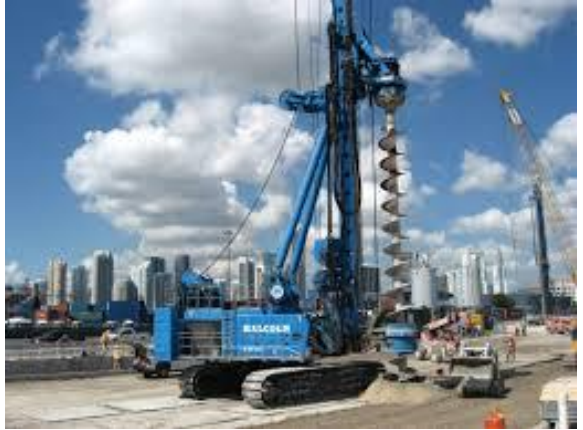
Continuous Flight Auger Installation
