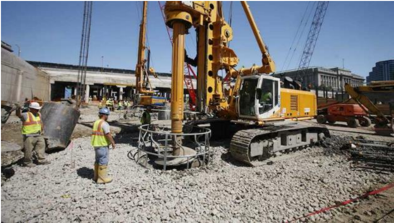
Safe ground conditions for equipment
