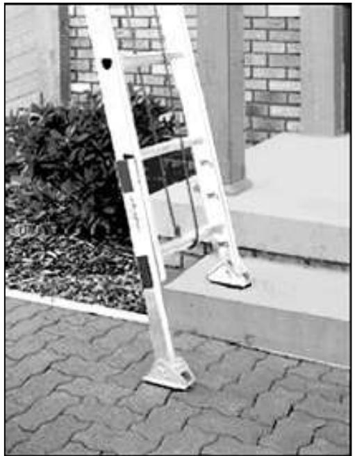
**Use a wood or plastic wedge or a ladder leveler leg when using ladders on uneven surfaces.**
