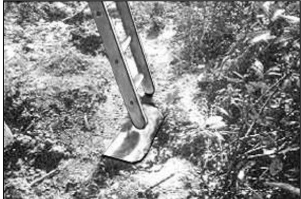
**Over half of all ladder accidents are caused by falls when the ladder tips over as a result of poor ladder placement.**
