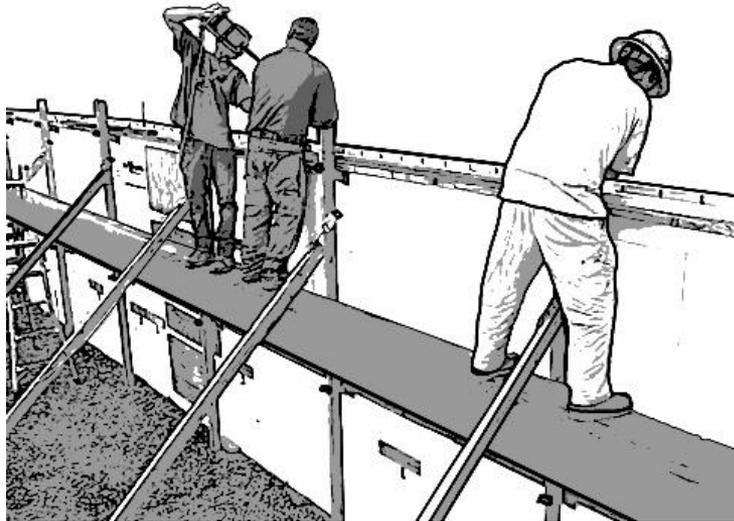
When forms are removed, it is important to determine if the walls need to be braced.
