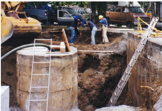
Manhole in Excavation
