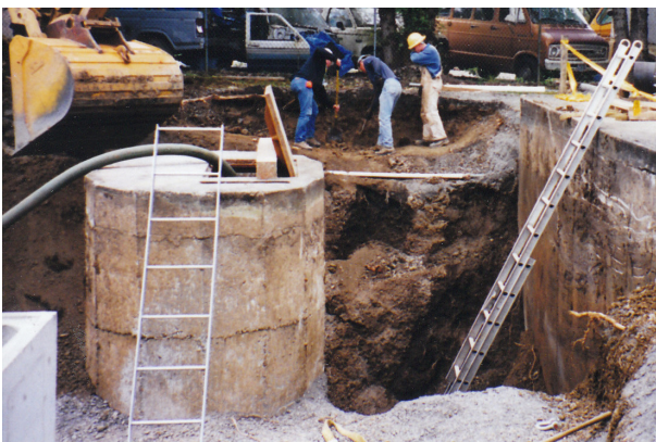
Manhole in Excavation
