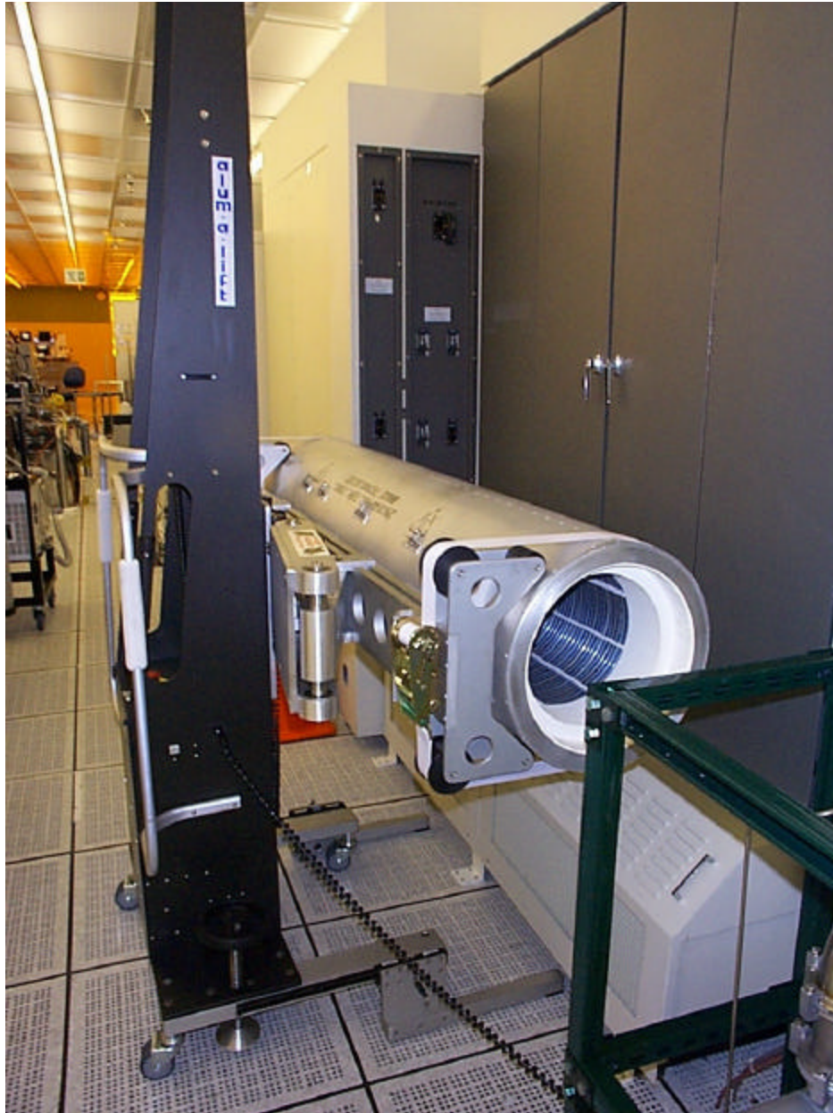
Hoist with heater core attached and ready for installation
