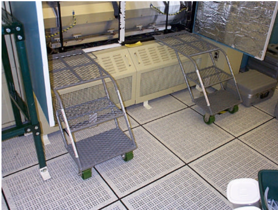
Elevated work platforms dedicated to the core change process. Note the space between the platforms for the hoist
