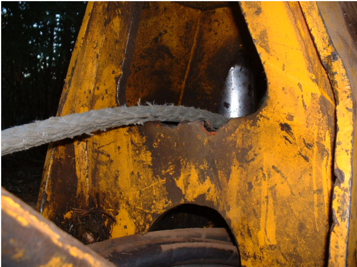
Figure R29. Gouges cut into ½-inch plate steel by poor operating practices with steel wire rope create cutting edges detrimental to synthetic rope longevity.
