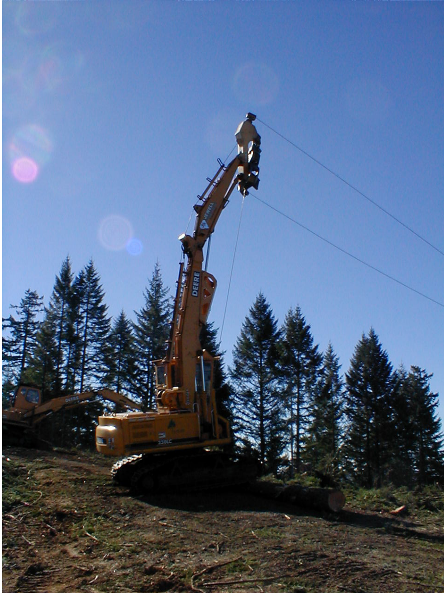
Figure R21. “Yoader” configuration used with one field trial of synthetic lines for rigging straps, guylines, and support jack lift lines.
