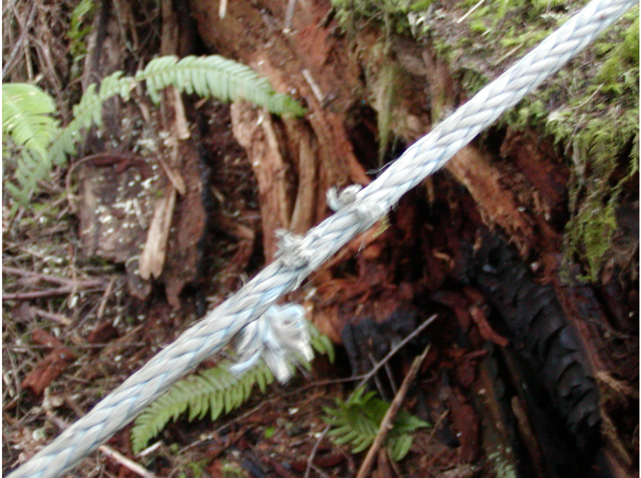
Figure 48. Tail tree guyline with partial cuts in a couple of non-adjacent strands. While this situation does not exceed manufacturer's out of service criteria, removal of this section would be a prudent action by the operator.
