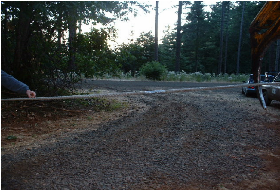
Figure 38. Synthetic ropes may be quickly and cleanly long spliced to repair a damage section or lengthen an existing line. The duct tape section identifies the crossover point of the long splice. The operator's finger and the grapple arm are the approximate terminations of the buried tail to create the entire long splice in this 3/4-inch diameter synthetic winch line.
