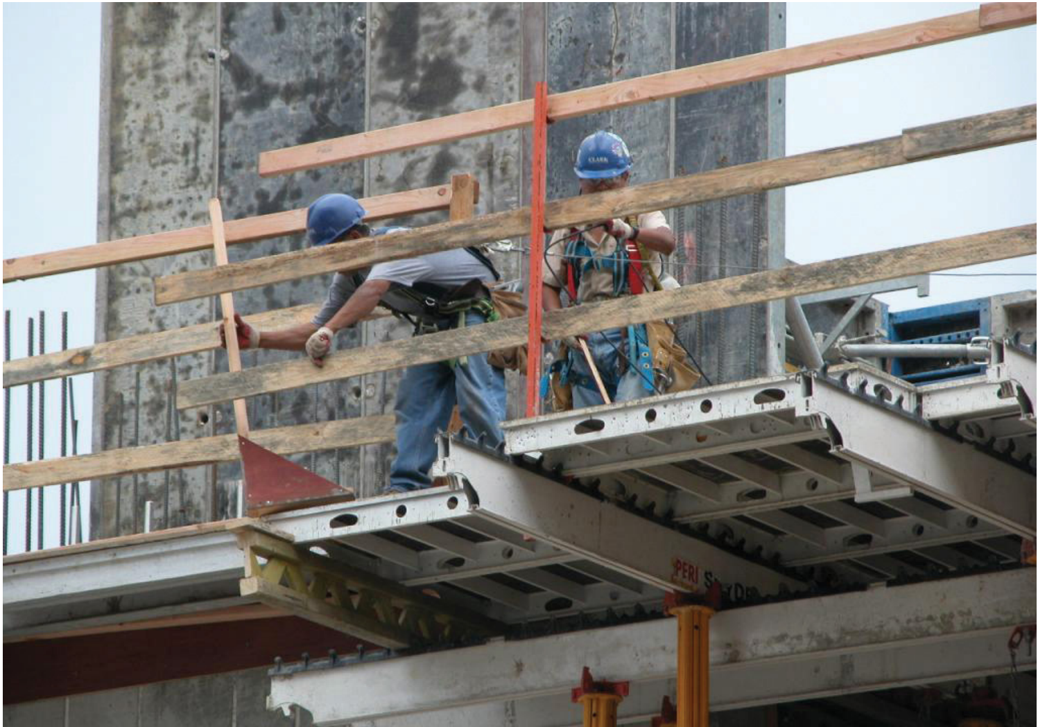
Assembling guardrails. Worker at leading edge tied off to a retractable lanyard.
