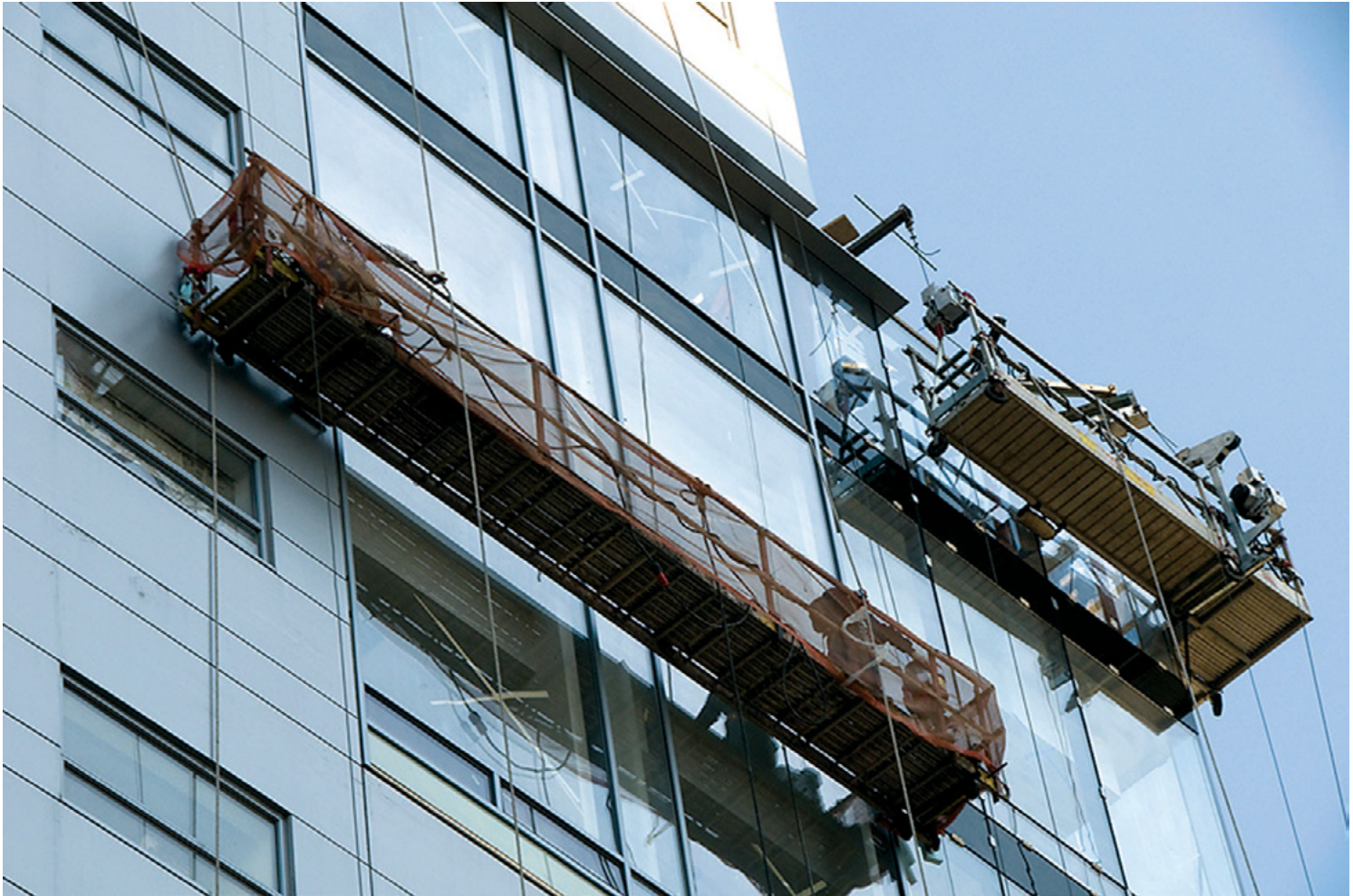
Adjustable suspension scaffolds.
