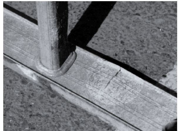
Equipment inspections are critical. Do you see the small fracture in this picture?
