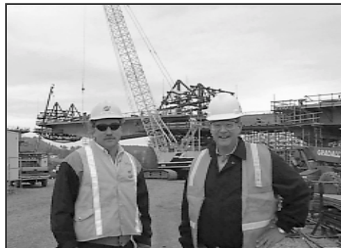
Walker Kimball and Peter DeLuca visit the construction site.
